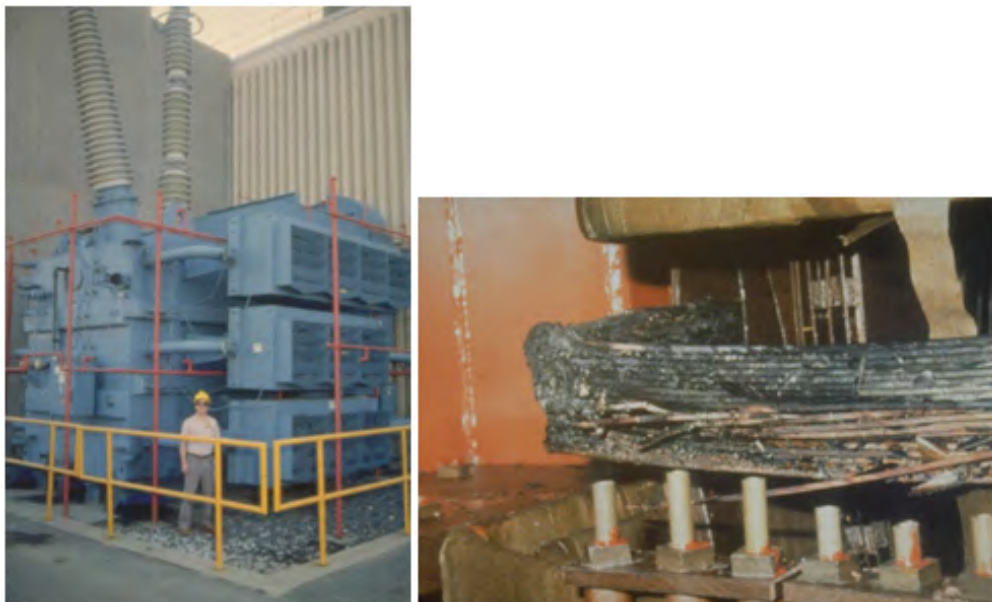
Transformer at the Salem Nuclear Plant, damaged by March 1989 solar storm[4].
